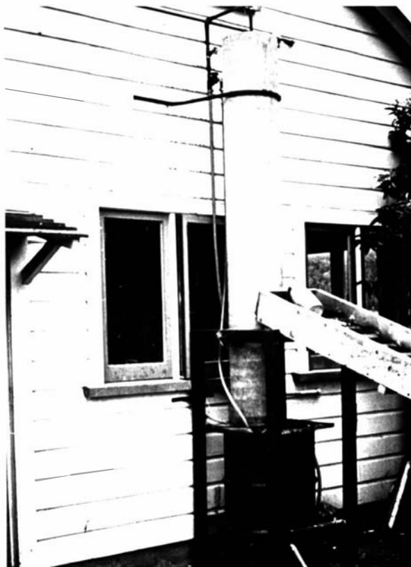
PLATE 4:1 Single 195 litre tank and trickling filter unit.
