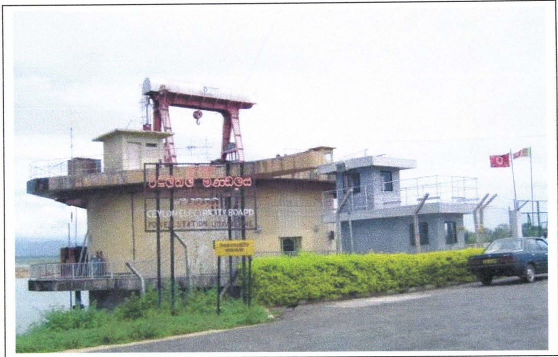
Fig. C.1: The left bank Udawalawe power station in which 2 out of the 3 turbines are located (Courtesy: Ms Hemali Senevirathne, present engineer in charge at Udawalawe)
