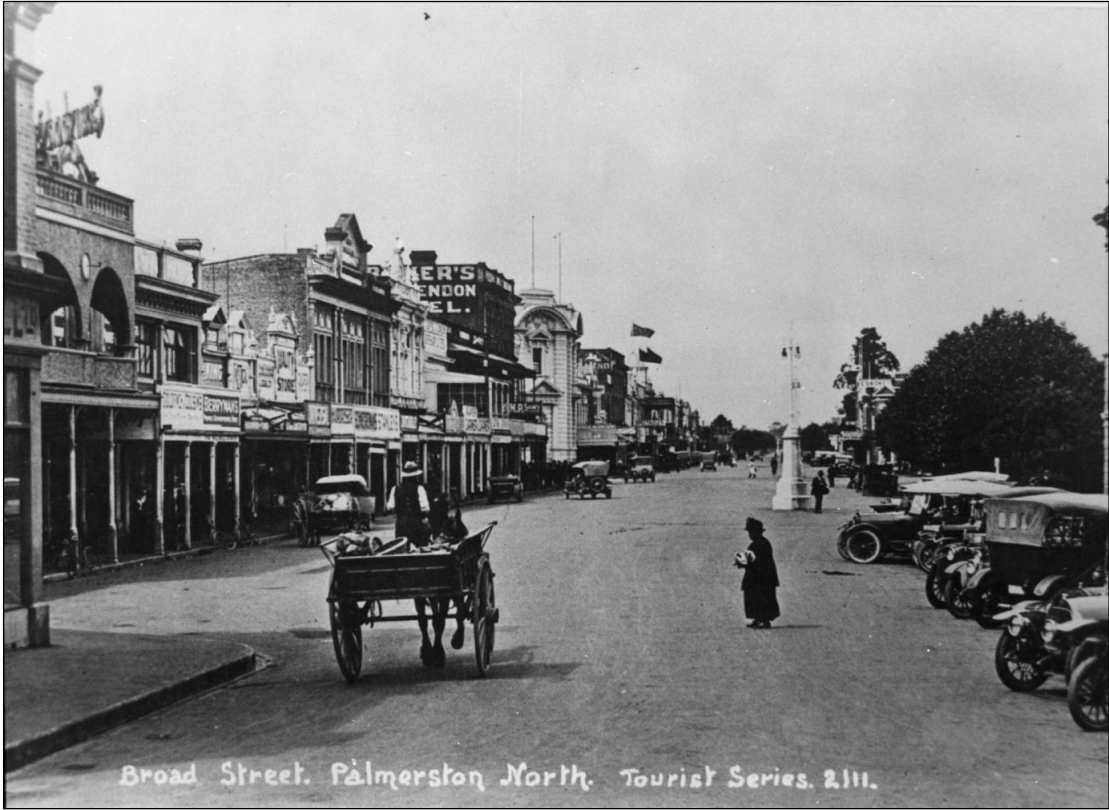
Image 3: View from George Street into Coleman Place and beyond (into The Square and Broad Street), circa 1925. 60
