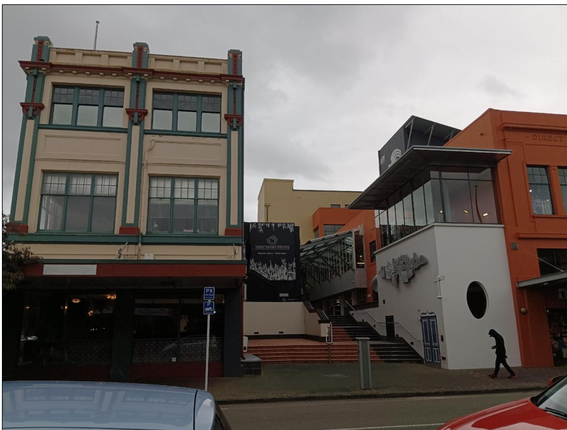
Image 34: A view from George Street showing the much smaller former CM Ross building (on the corner with Coleman Place) after its partial demolition, with the creation of the Palmerston North City Library's entrance walkway. 464
