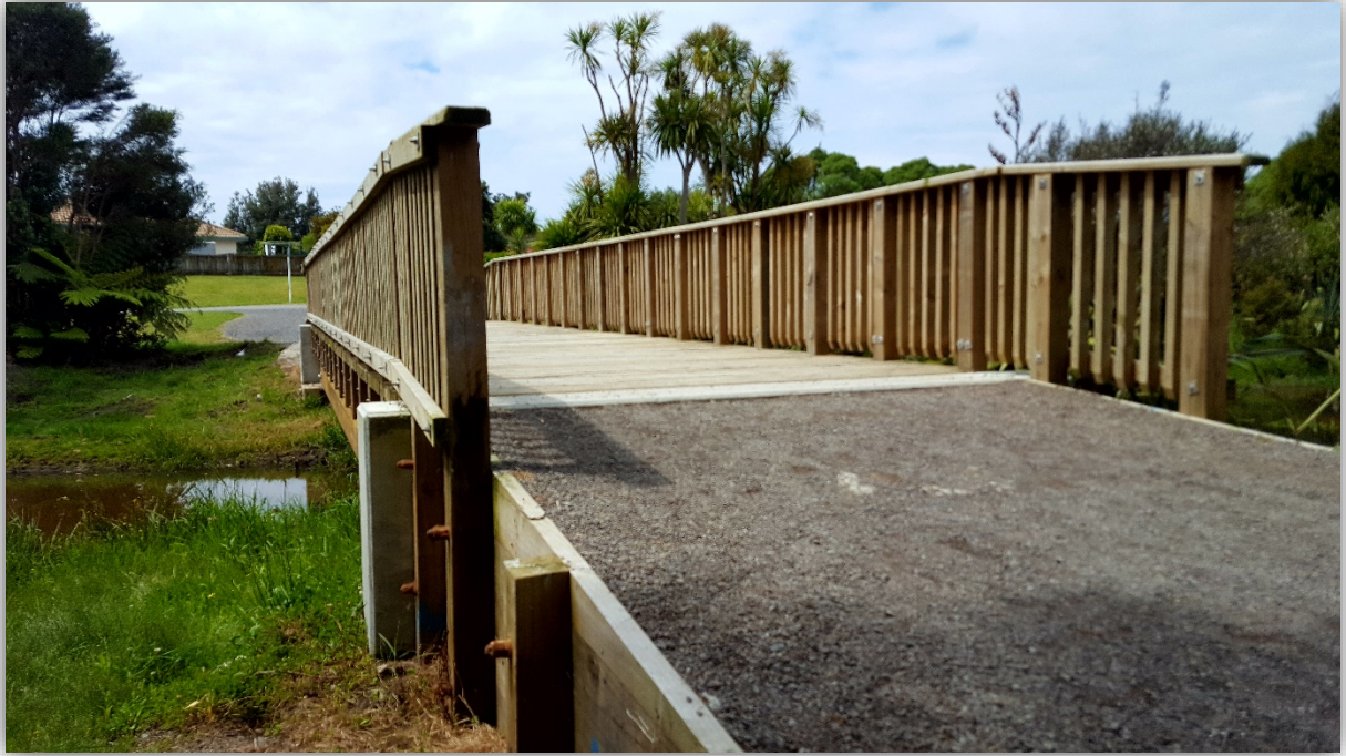
Pāpāmoa Evacuation Bridge
