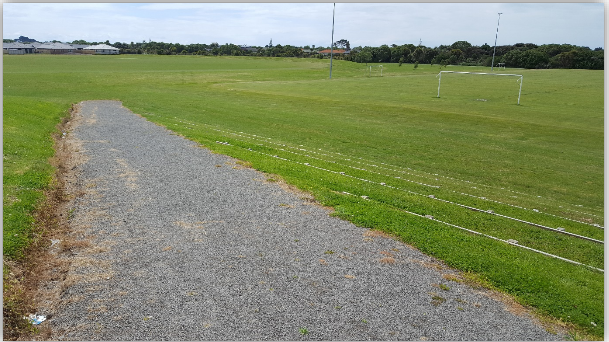
Pāpāmoa vertical evacuation mound (Bell Road)
