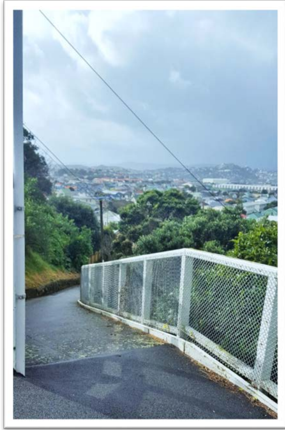
An evacuation walkway above Lyall Bay
