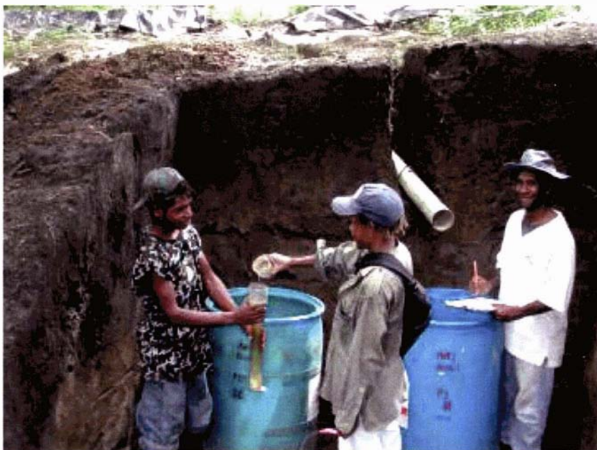
Plate 4.6 Runoff collection pit. Note shelter not yet built over
