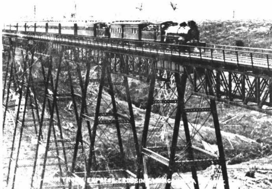
PLATE 11 - Mangaweka Viaduct: North Island Main Trunk Express crossing viaduct in early twentieth century.
