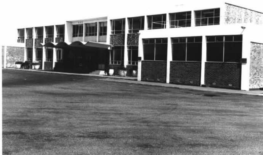
PLATE 19 - Palmerston North Railway Station, 1971: Tremaine Avenue location.
