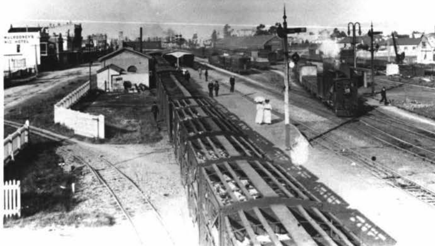
PLATE 18 - Palmerston North Railway Station 1910: the station remained on this site until 1963 when facilities were moved to Tremaine Avenue. Note the stock wagons. The railway at this stage was an important transporter of livestock.
