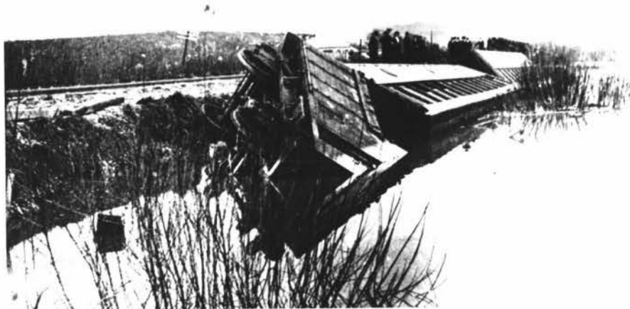
PLATE 8 - Train derailed in Makerua Swamp: this photograph taken in either late 1880's or 1890's. Note the undrained swamp land.
