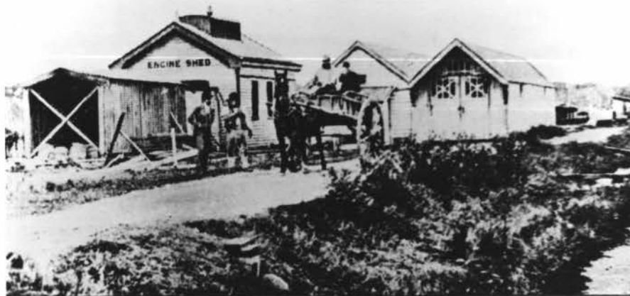
ENGINE AND TRAM SHEDS, PALMERSTON NORTH 1877. Formerly Situated opposite the present Court House.
