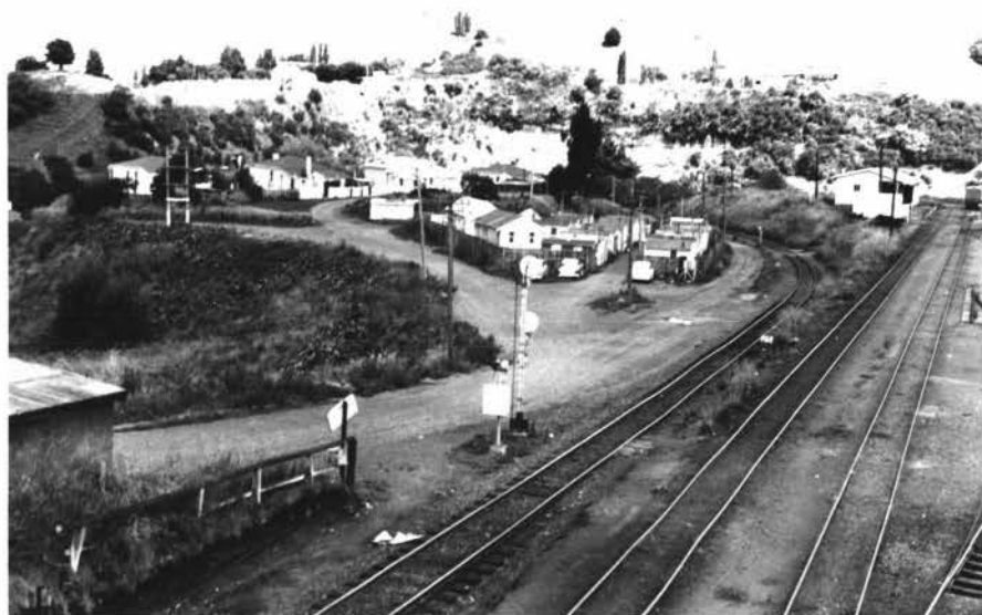
PLATE 24 - Single Men's Huts, Railway Compound Taihape, 1971. Photo: K.G.T.
