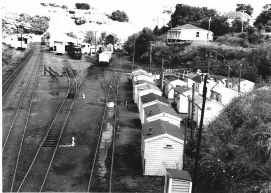
PLATE 25 - Single Men's Huts, Railway Compound Taihape, 1971. Photo: K.G.T.
