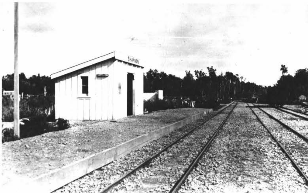
PLATE 5 - Shannon Railway Station: this photograph probably taken in the late 1880's or early 1890's. Note the dense strands of timber in close proximity to the town.
