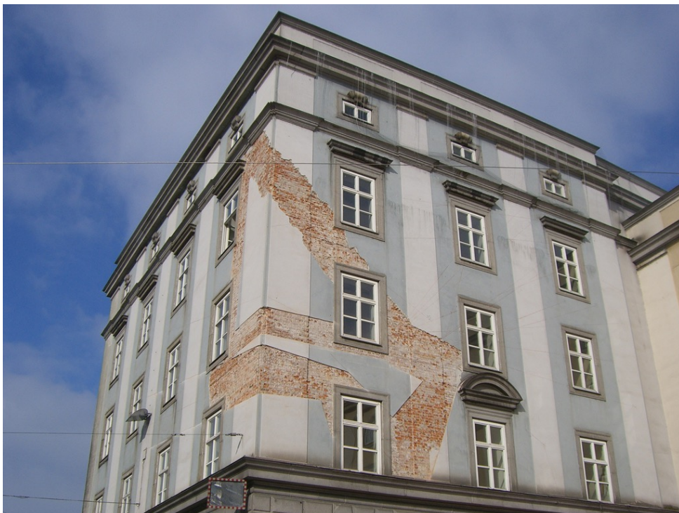
Figure 13. Hito Steyerl and Gabu Heindl Architecture, Der Bau (The Building), Linz, Austria, 2009. Photograph by Gabu Heindl. (Courtesy of Hito Steyerl and Gabu Heindl.)
