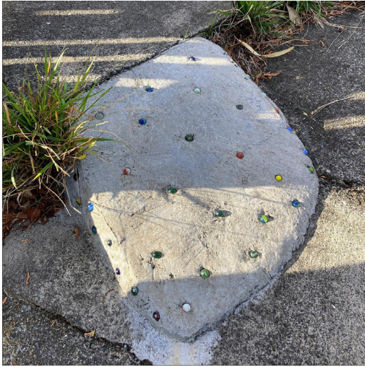
← Fig. 25. Cement ramp on Lavaud Street, Berhampore, 2022
