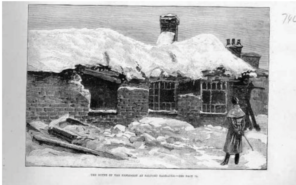
Figure 4.1: Salford Barracks bombing on 14 January 1881 showing damage to the meat shed from the barrack's side 14 .
