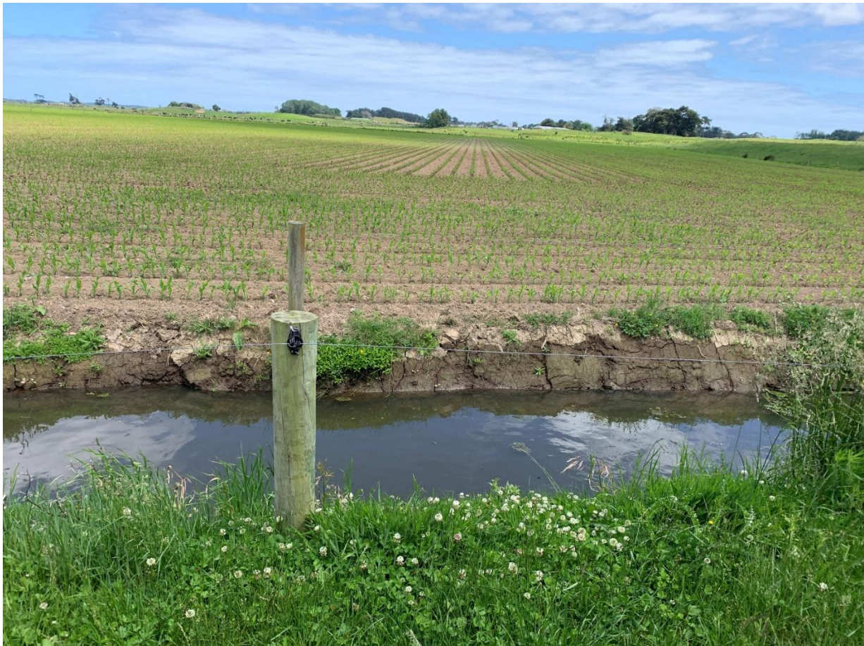
Figure 40: Controlled drainage in operation during summer season, with artificially-elevated drainage water effects seen in the soil profile moisture at this drain cutting. Taken November 30, 2023 near PCD-1 site.
