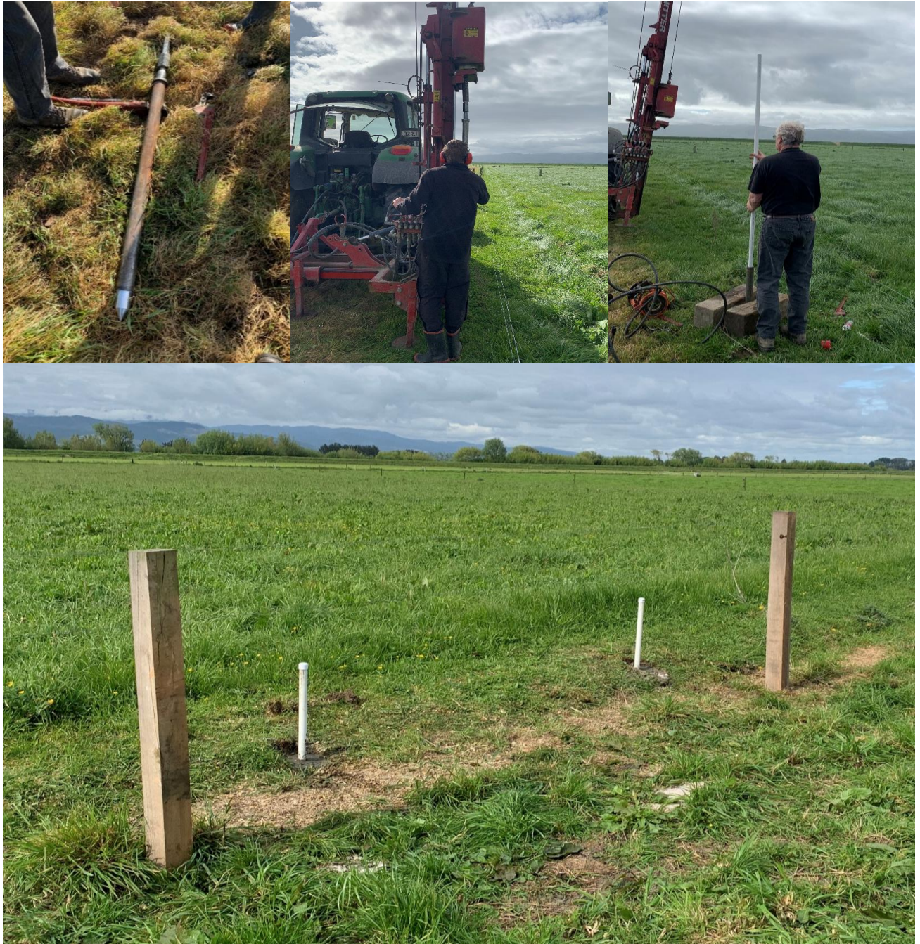
Figure 12: Installation methodology of piezometers illustrated. Top left: steel casing with driving point used to create space for piezometer; top middle: steel casing being rammed in with post rammer; top right: piezometer being inserted into hole; bottom: piezometers at completion of installation.
