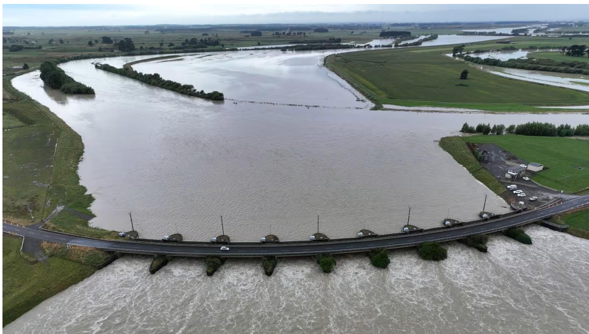
Figure 6: Moutoa sluice gates in operation. Water flowing from the flooded Manawatu River mainstem (mid- and background), into the floodway (foreground) via the sluice gates (Baalbergen, 2024).
