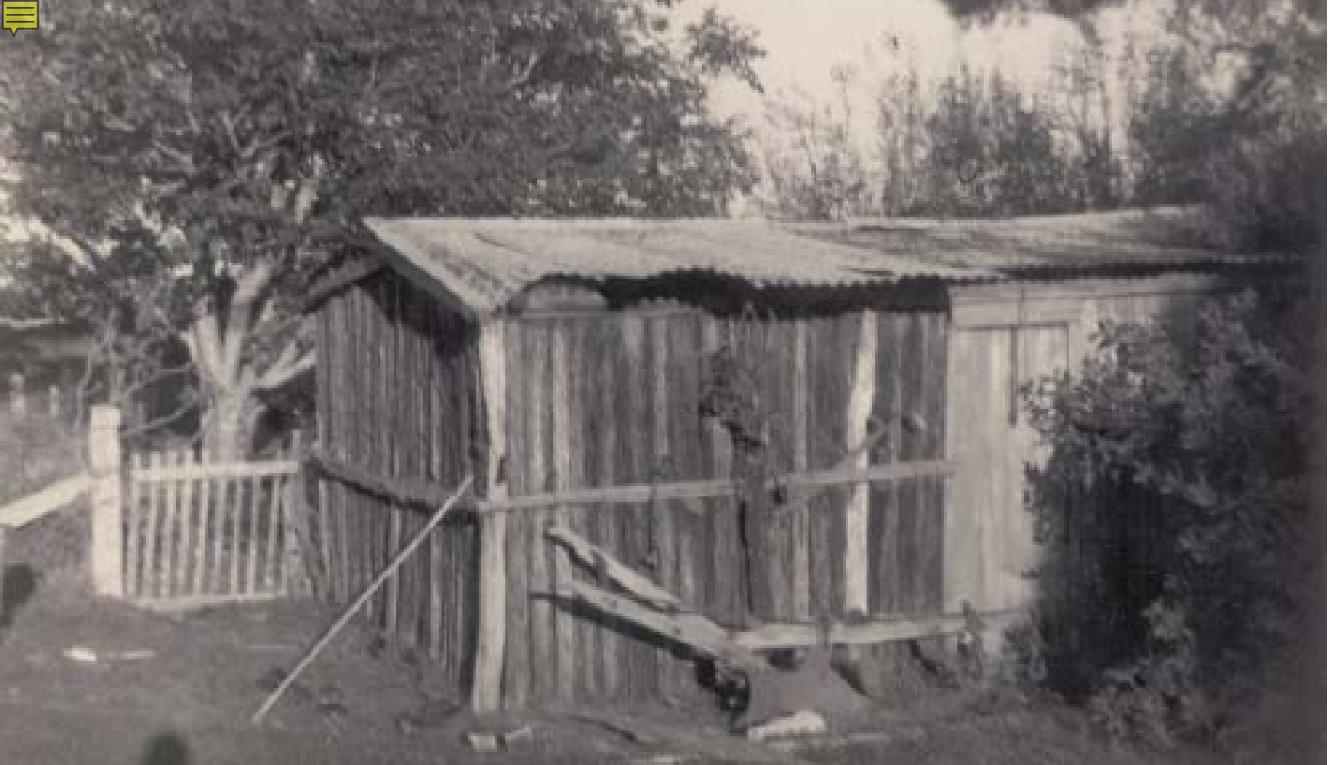
Log cabin 6m x 4m built from stems of “ponga” tree ferns. James Morgan lived here c. 1920 – 1945 until he married. Note horse drawn plough used by James for pasture establishment and rabbit traps which provided income during the great 1930s depression.
