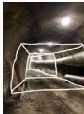
Figure 17: Backfilling of the Pilot tunnel on sketch, this relates to Figure 13.
