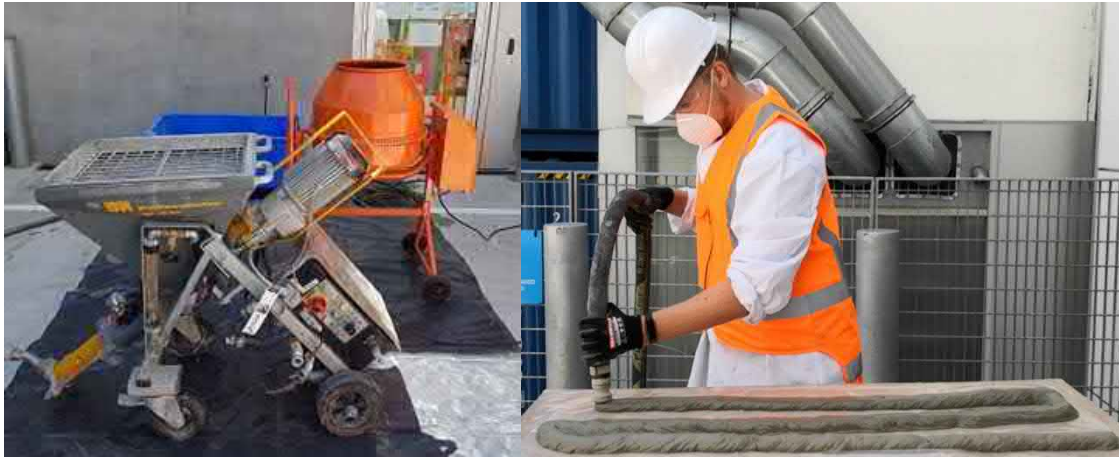
Figure 5 – (Right) Concrete mixing and pumping machines used in this research, (Left) Concrete consistency and flow test for calibration of the pumping speed.
