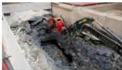
Figure 18: Mercury station box structure team excavating into the pilot tunnel, this relates to Figure 14.
