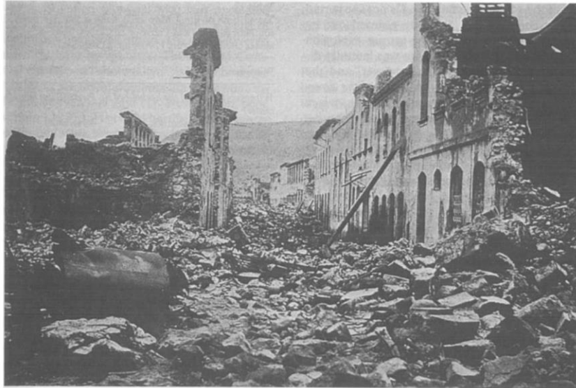
Figure 2.2: Photograph of the Rue Victor Hugo in the town of Saint Pierre (Martinique) after the passage of the deadly lateral blast PDC in 1902. From Tanguy 1994.
