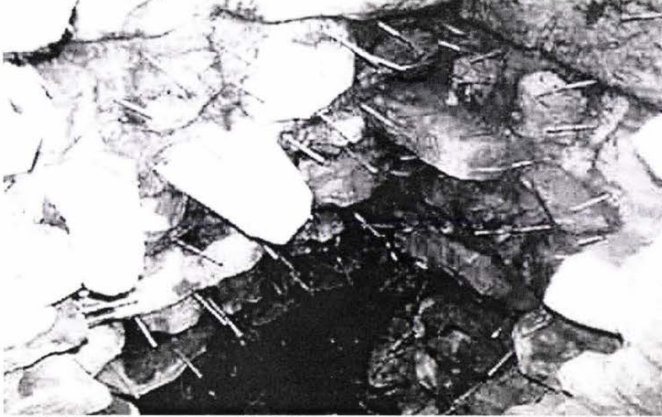
al-Ka'abah's interior walls being strengthened in 1957 CE (1377 AH)
