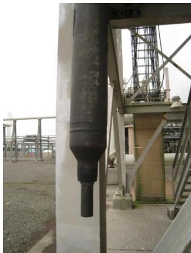
Figure 9.2 Specimen Reformer Tube Extraction End
