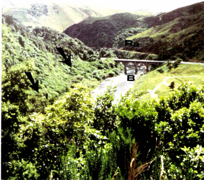
Plate 2, Engineering structures in the Manawatu Gorge showing the main trunk railway (Ra) line, State Highway bridge (B) and the Ruahine Fault trace (arrows)
