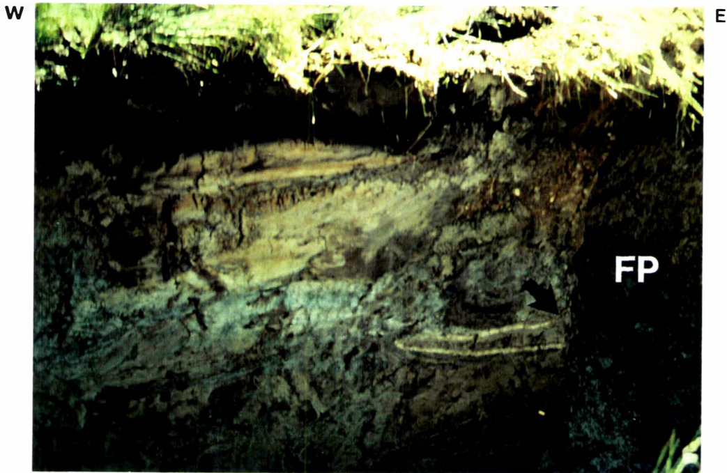
Plate 34, The Wellington Fault plane in the McCool 1 trench, north wall. Tephra (arrow, aged between 5206 \pm 81 yrs and 805 \pm 58 yrs B.P.) terminate abruptly against the fault plane (FP) which lies to the west of the tephra (Figure 23). The fault plane is composed of silty clay with pebbles (fault gauge).
