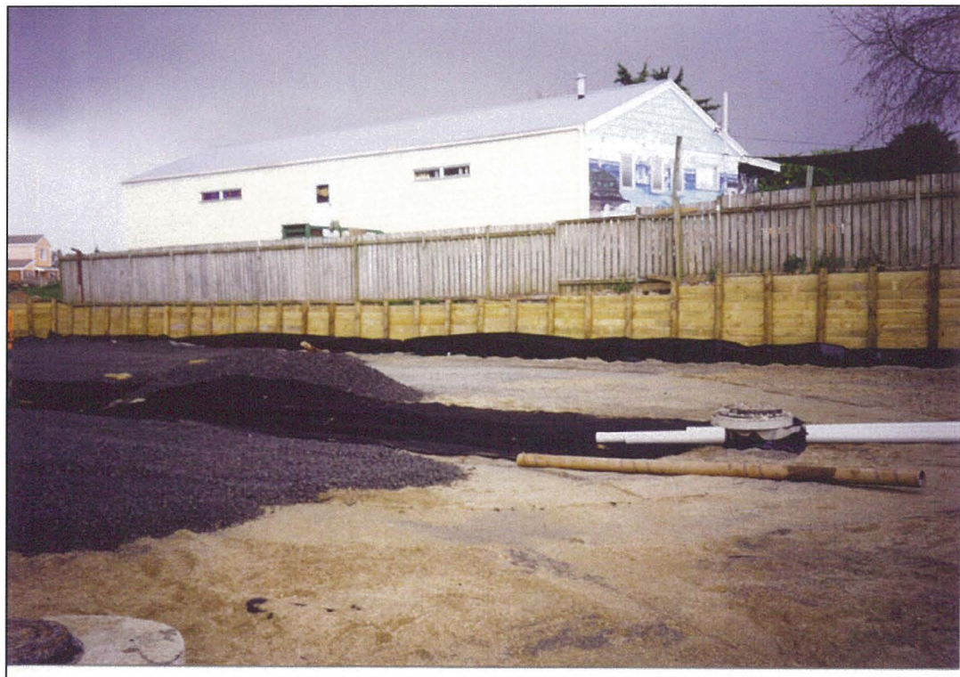
FIGURE 3.22 CENTRAL AREA UNDER CONSTRUCTION
