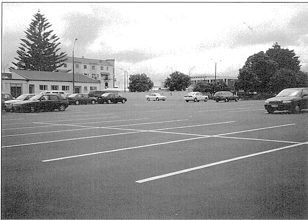
FIGURE 5.10 PAPATOETOE WARD OFFICE CARPARK
