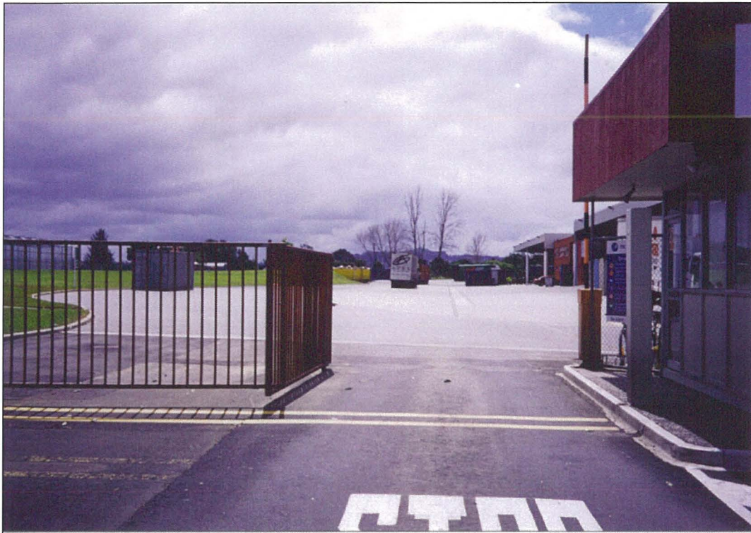
FIGURE 5.13 PROGRESSIVE ENTERPRISES TRUCK YARD
