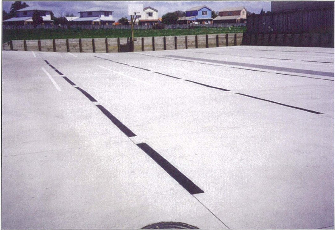
FIGURE 3.23 CENTRAL AREA BEING CONSTRUCTED
