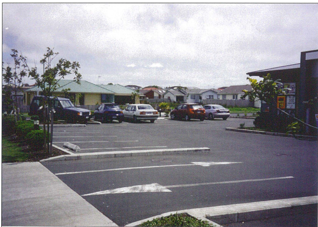
FIGURE 5.15 PHARMACY CAR PARK
