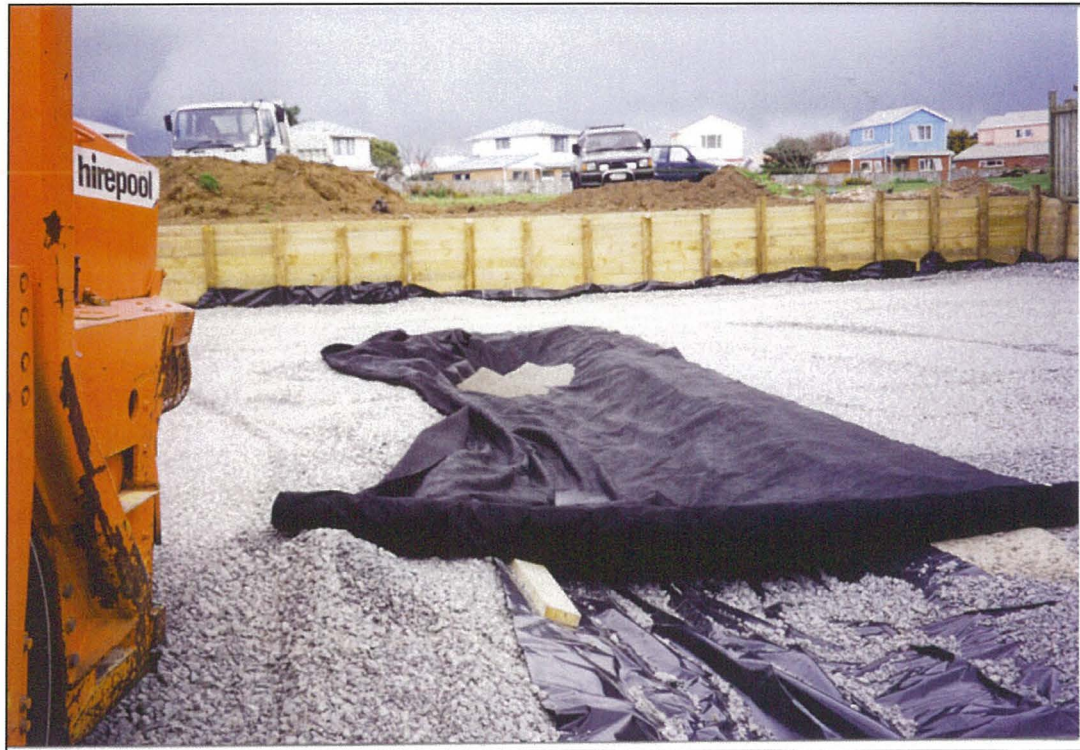
FIGURE 3.24 CENTRAL AREA COMPLETED.
