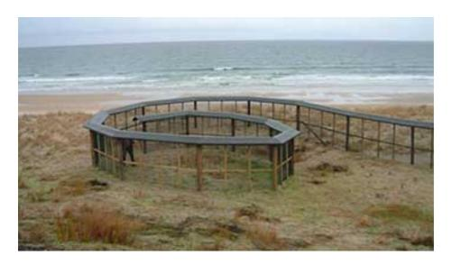
Plate 5. 'Koru' shaped ends of Xcluder predator proof fence used at both Tawharanui and Cape Kidnapper's (Xcluder Pest Proof Fencing Ltd, 2010).
