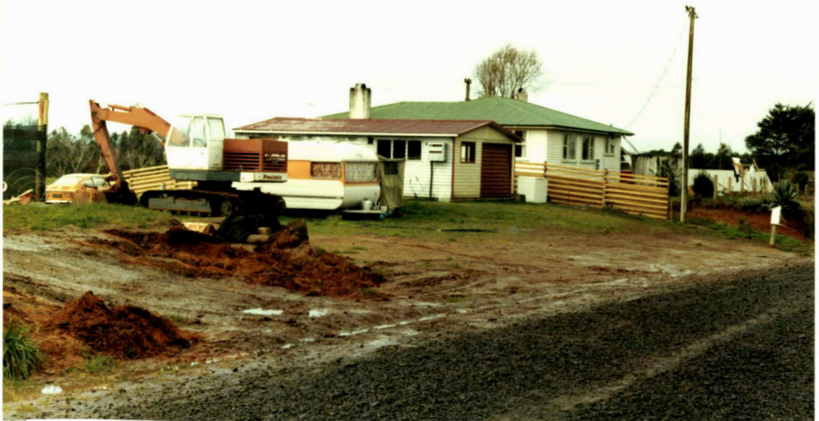
b Existing Dwelling and House Site being Prepared
