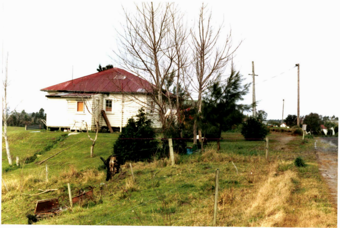
a Substandard Dwelling, to be Removed
