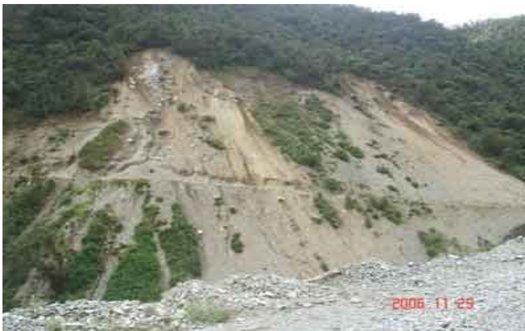
Figure 2.10 Erosion caused by mining activities in the watershed
