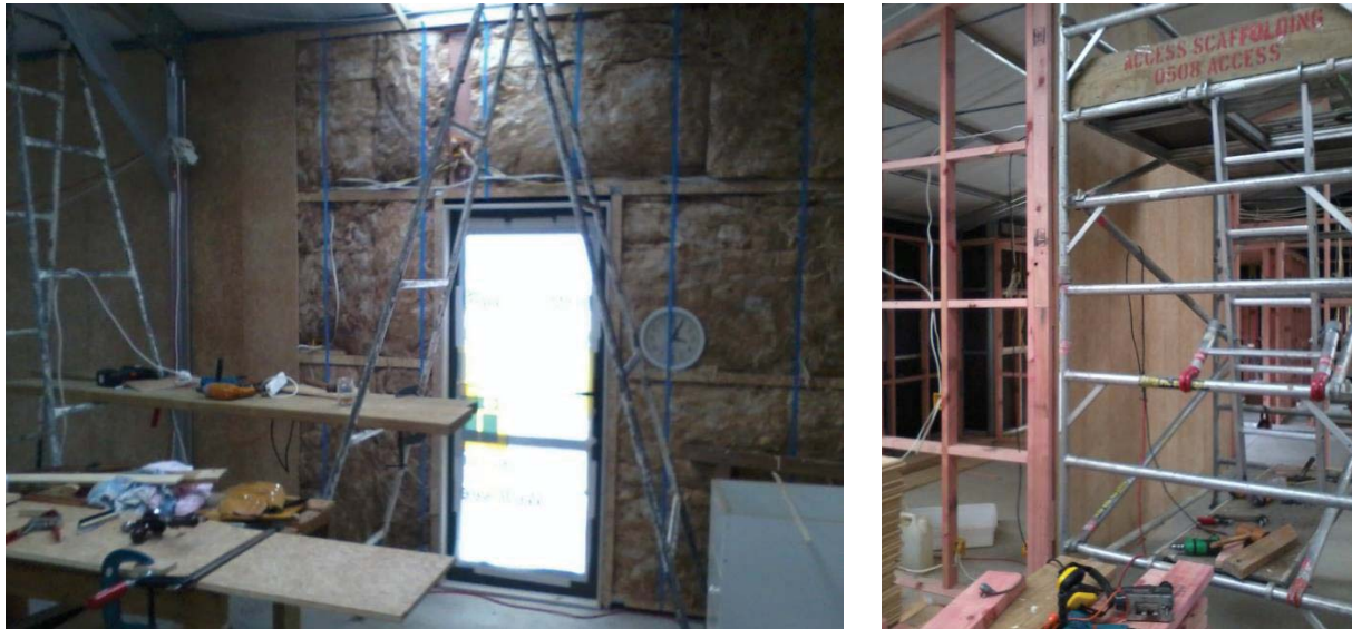
Figure 6. Various forms of scaffolding used to construct the internal Shed
