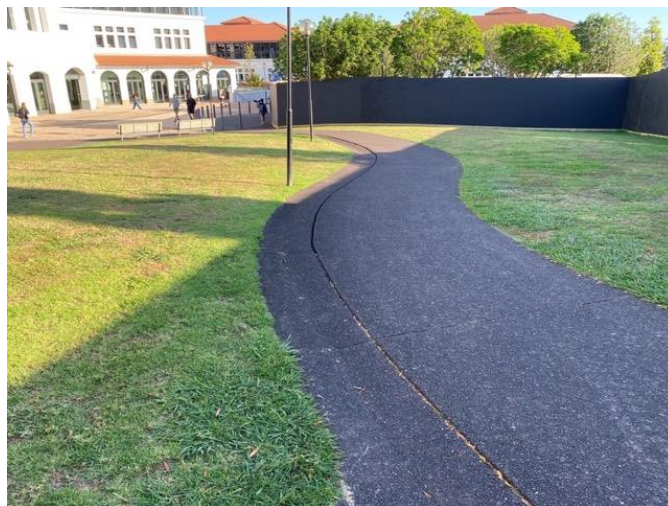
Figure 13: A curved ramp near the Atrium Building.
