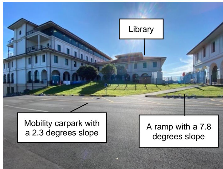
Figure 12: The mobility carpark near the library.
