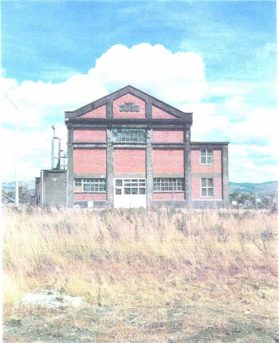
Photo 8. A more recent view of the Power Station, 1970s or 1980s.
