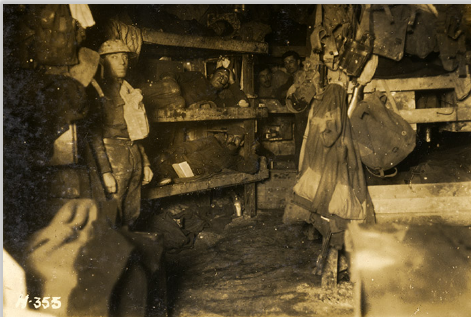
The night shift of the New Zealand Tunnelling Company in their bunks below ground (PH-ALB-419-H355) 1 .
