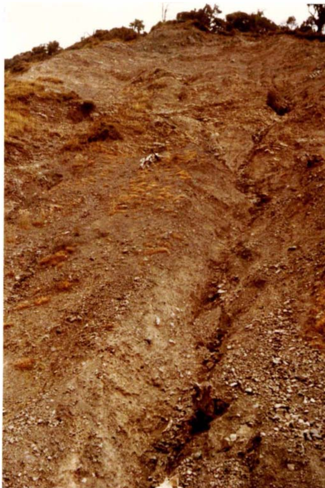
FIGURE 10.21: Rilling within colluvium at the head of a debris slide scar. Note how the smaller rills near the top of the scar merge further downslope into a single master rill. Photograph taken in Otamarahu catchment at locality T23/612107.
