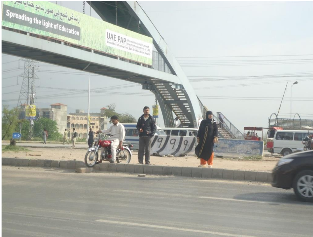
Figure 7. 10: People crossing road instead of using the overhead bridge
