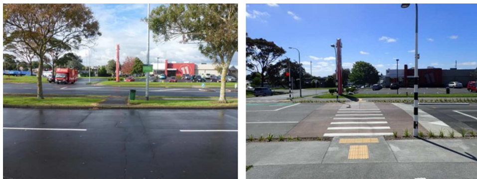
Figure 3. Mascot Avenue before and after raised table pedestrian crossing instillation creating pedestrian access to the Town Centre.
