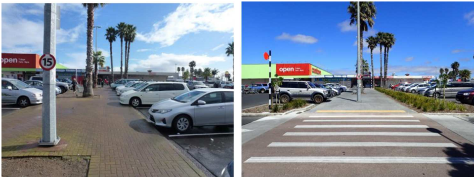
Figure 5. Town Centre on Mascot Ave before and after raised zebra pedestrian crossing instillation through carpark.
