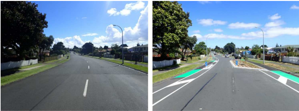
Figure 8. Friesian Drive before and after the instillation of chicanes, cycle lanes and the removal of parking. These changes narrowed the street to slow cars down, making it safer for pedestrians.
