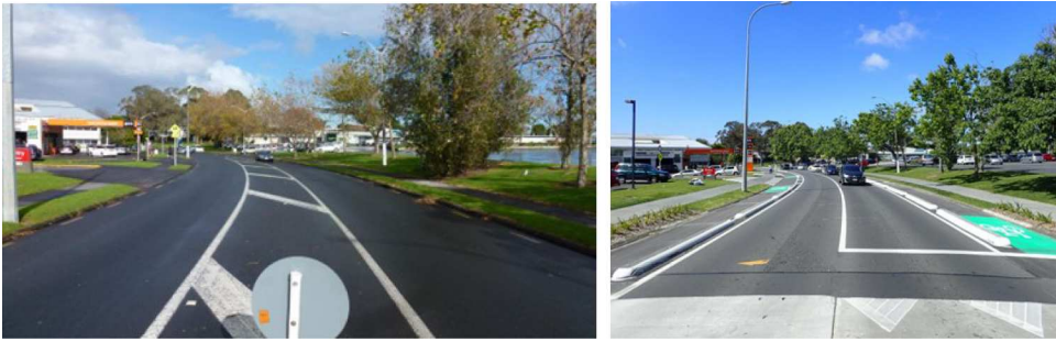
Figure 7. Mascot Avenue near the Town Centre before and after on-road bike lane instillation. Separated cycle lanes have been installed on both sides of the road, making it narrower, meaning that cars move slower. In addition, the footpath has been upgraded and there is a raised crossing in the foreground.
