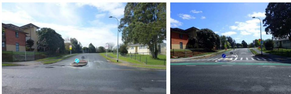
Figure 2. Intersection of Mascot Avenue and Friesian Drive before and after instillation of a painted zebra crossing for pedestrians. In addition, a painted bicycle lane with plantings alongside it has been included.
