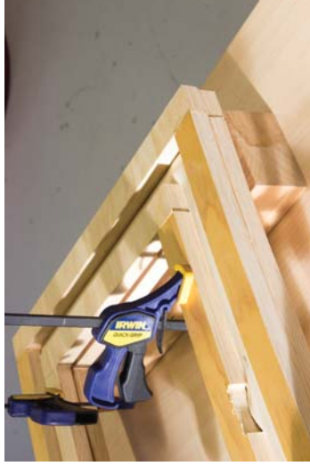
Figure 271 Plywood jigs were used to maintain the shape of each component while injecting the cavity with expanding foam.
