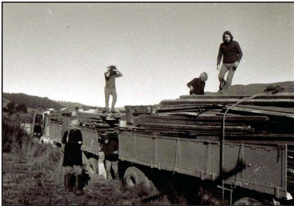
Unloading the demolition timber for the community house.
