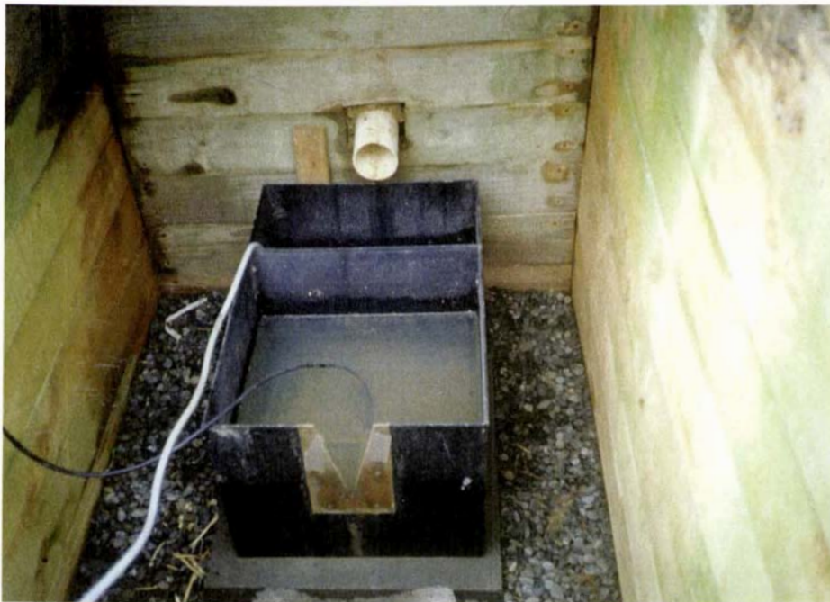
Fig. 2.3 V-notch weir for monitoring the flow rates
