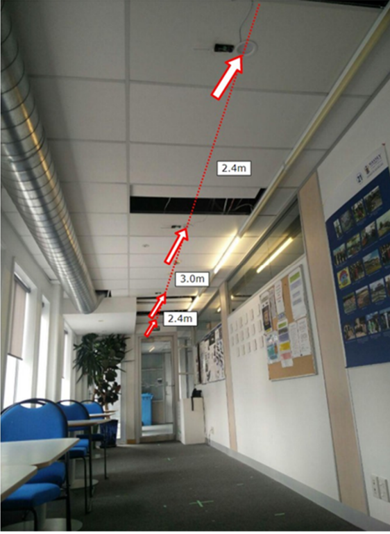
FIGURE 2. Anchor Nodes Installed in Hall
