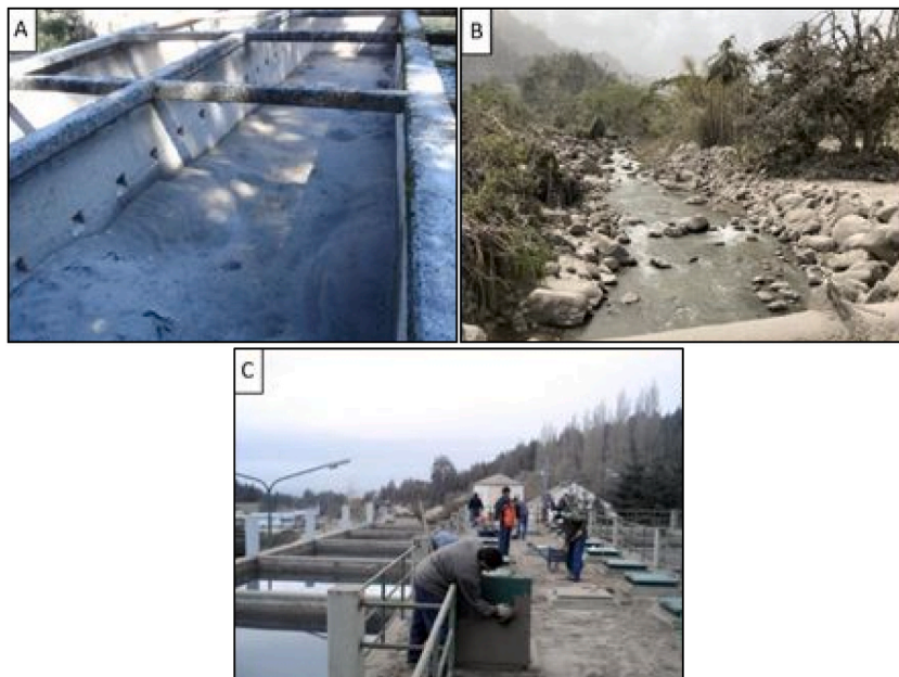
Fig. 2. Direct impacts from volcanic ashfall to water supply. A: Ash inundation in settling ponds in a stream-fed water treatment system in Argentina following the 2011–2012 Puyehue-Cordón Caulle eruption (Photo Credit: Carol Stewart). B: Thick ash deposits surround the Richmond River near water intakes, St Vincent during the 2021 eruption of La Soufrière (Photo credit: UWI Seismic Research Centre). C: ~50 mm ashfall at Bariloche WTP following the 2011–2012 Puyehue-Cordón Caulle eruption (Photo credit: Departamento Provincial de Agua, Bariloche).
