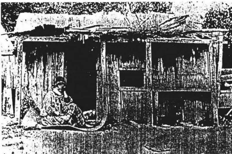
1.3- A slab whare with chimney and a bark roof, King Country, early 1900s.
