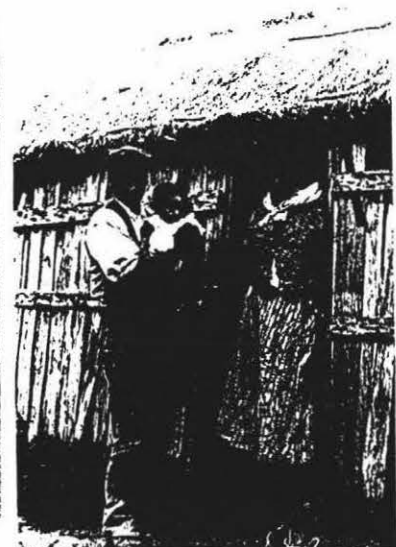
1.4- A paling house with a thatched muka roof, a kind common in the Hokianga district in the early 1900s.
