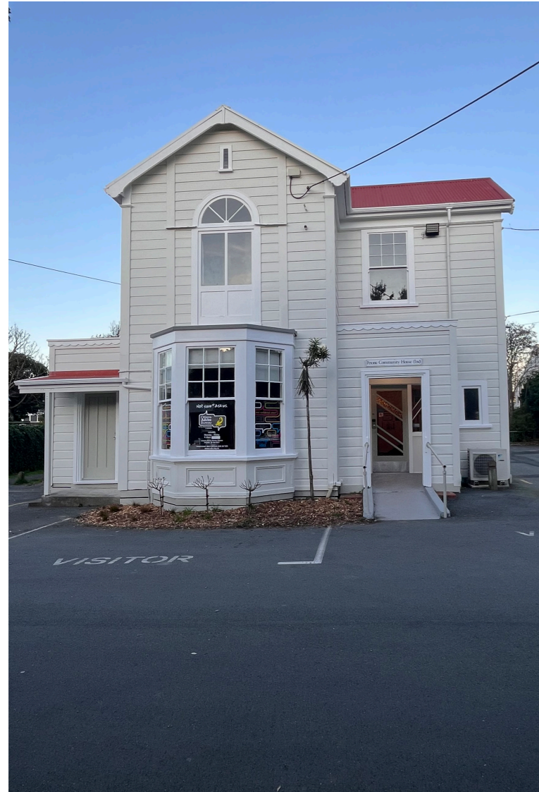
Fig 30: Front of Petone Community House, 2025
