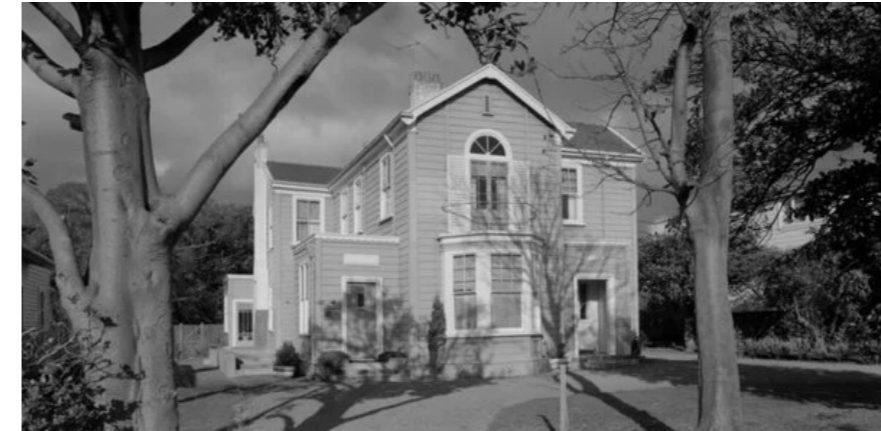
Fig 3: House at 6 Britannia Street Wellington, 1969
