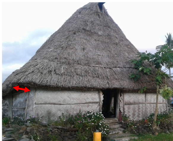
Fig. 19. Roof narrow extensions (eaves).
