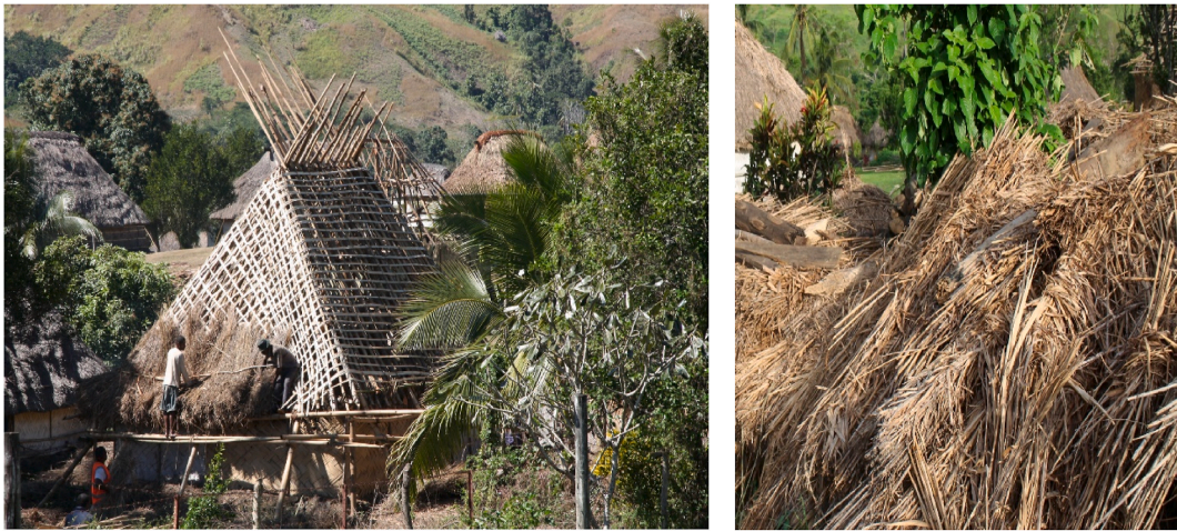
Fig. 14. Netting for the roof thatches (left); thatches ready in bundles (right) (Sources: Mark Heard, left; Author, right).
