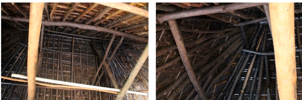
Fig. 15. Smoke fumigation of the house interior components.
