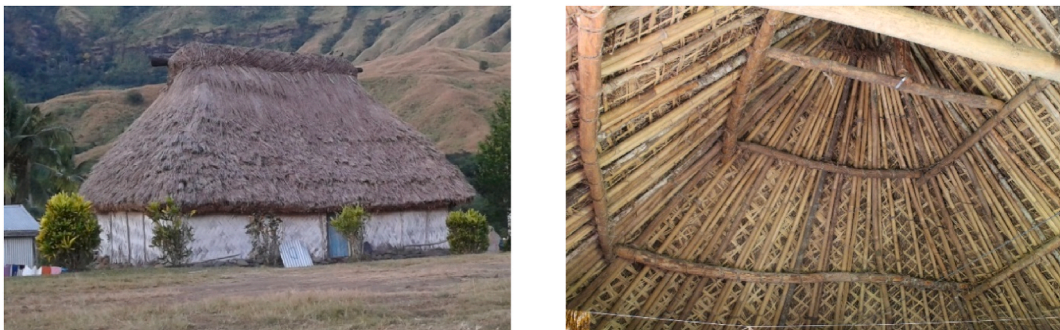
Fig. 12. Bure with the centre post from outside (left); bure without a centre post from the inside (right) (Source: Author).
