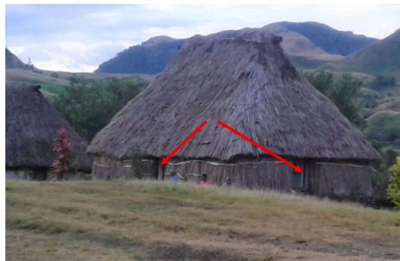
Fig. 21. House with thatched walls and roof and three short, narrow doors. (Source: Author).
