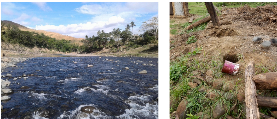
Fig. 7. Boulders from the river bed used for bure mounds (left); a bure mound with boulders, dirt backfill, and posts (right) (Source: Author).
