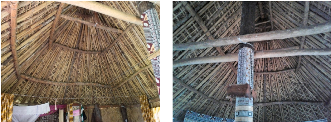
Fig. 9. Corner and wall posts, bamboo rafters and timber purlins (left); central post with crossbeam struts (right) (Source: Author).
