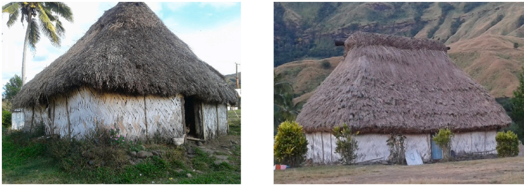
Fig. 8. (Small version) traditional bure without a centre post (left), (Large version) traditional bure with centre post (right).
