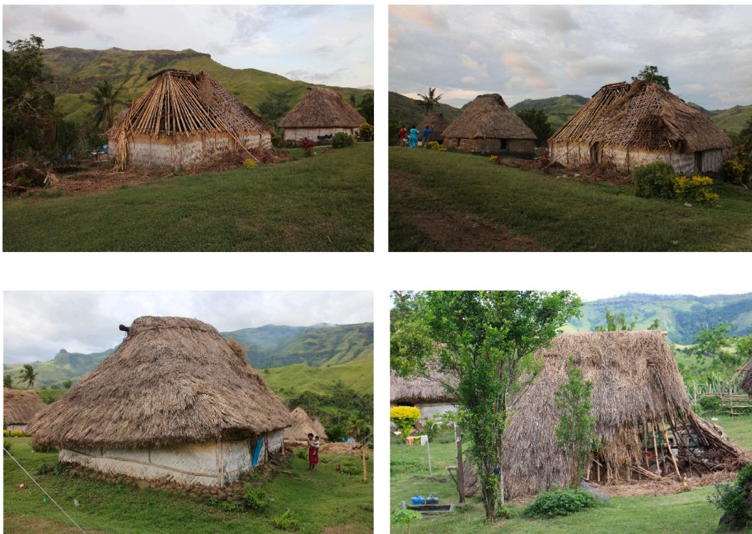
Fig. 5. Partially damaged bure houses, with only roof thatches destroyed (Source: The Author).
