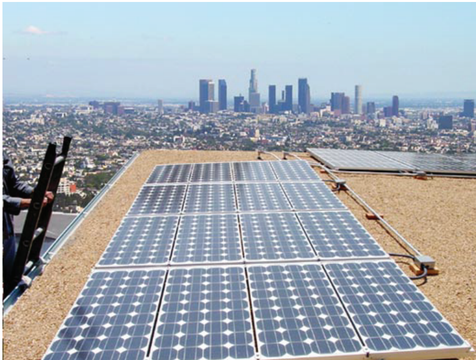
Figure009 “Los Angeles Solar Panels Installation”
