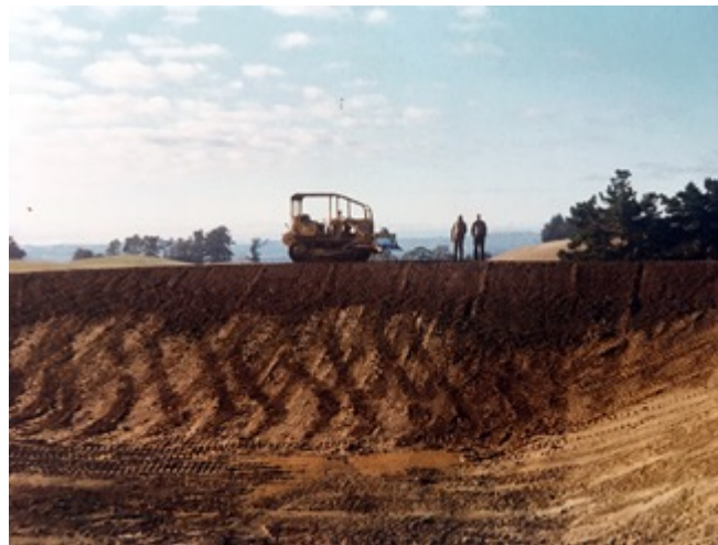
Fig. 5. My father and uncle at a dam excavation on Manawatū farmland near Feilding in the 1970's.
