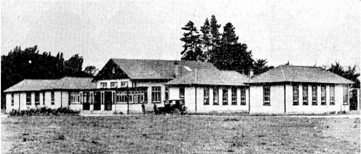
Figure 15: One of the self-contained villas at Templeton Farm School. This type of accommodation was thought to reduce the institutional aspect, and is very different in appearance to that of Seacliff. Press 10 Jan 1931, 17
