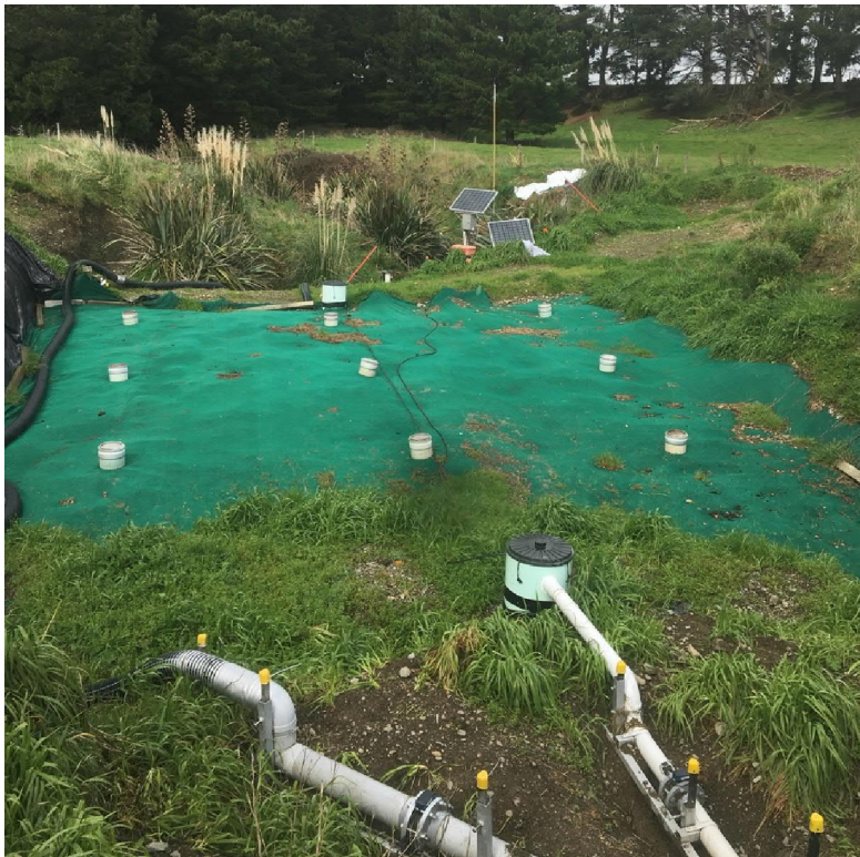
Figure 7. Denitrifying bioreactor set up (August 2022), (Photo taken by author).
