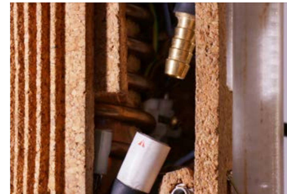
Quick disconnects were used for water hoses as well as one way valves to interrupt flow.
