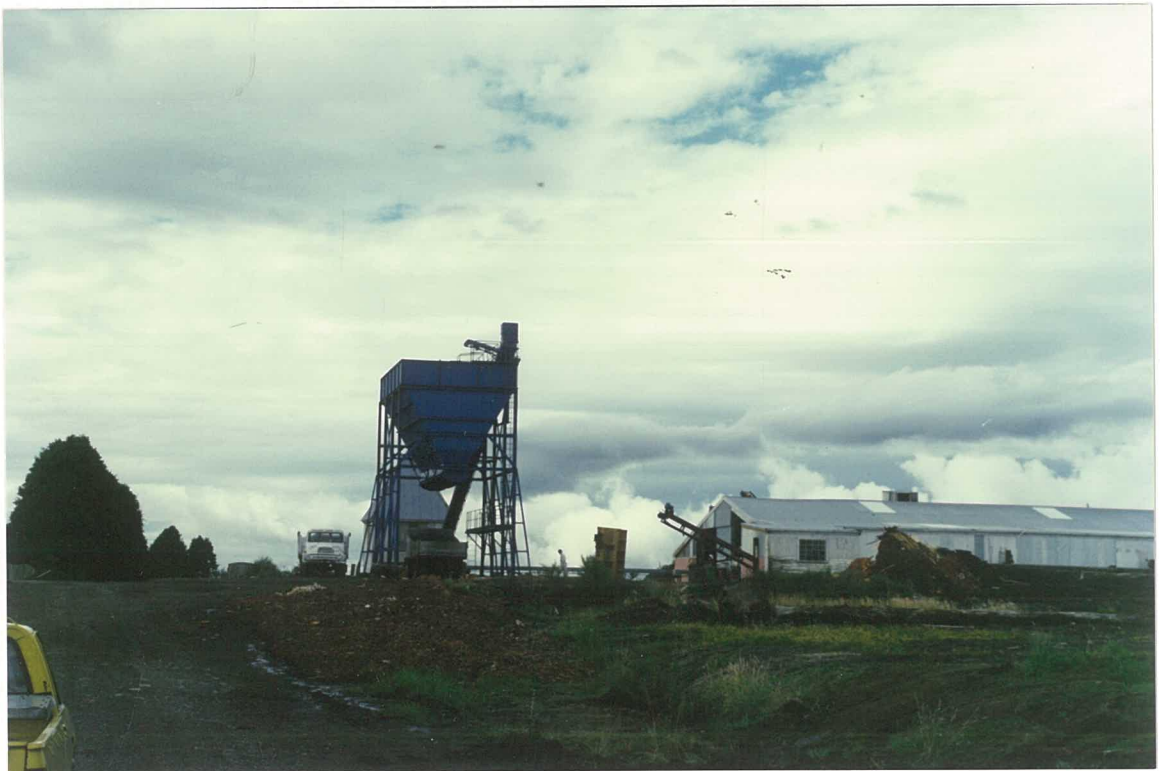
Figure 22 - Tongariro Timber Mill Hopper
