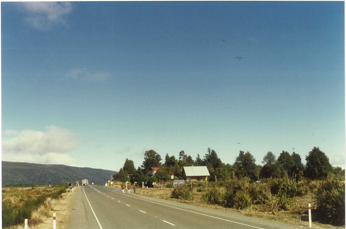
Figure 46 - State Highway No. 4
