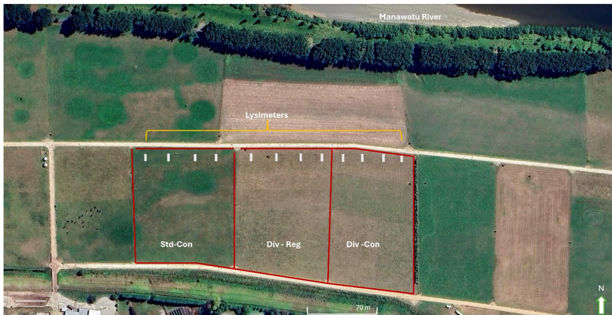
Figure 3.1: Experimental location and trench lysimeters located within each treatment paddock of the Whenua Haumanu study at Dairy 1 farm, Palmerston North, New Zealand. Aerial photo was taken prior to the establishment of the pasture treatments.
