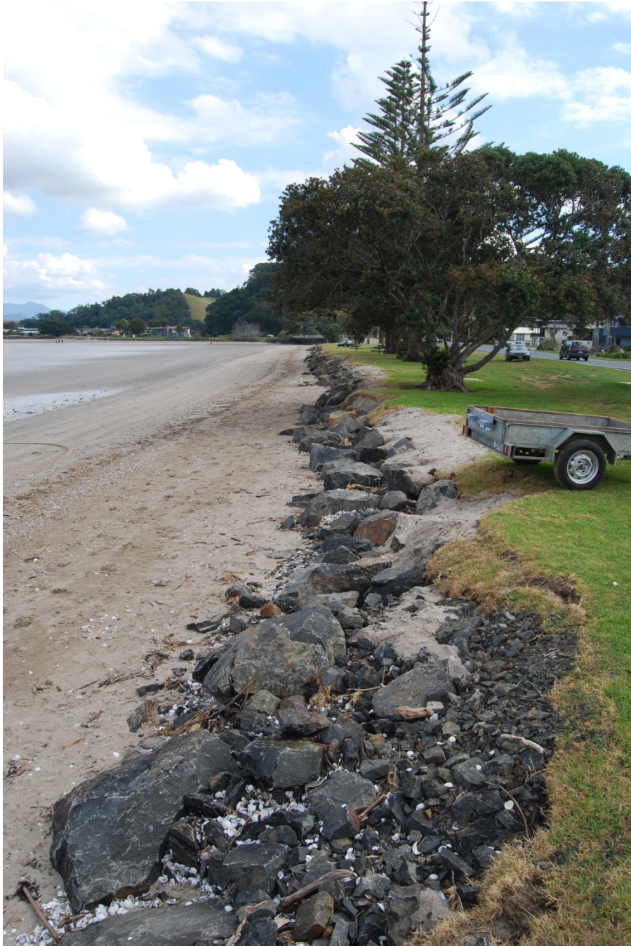
Figure 8.3: Short-term techno-fixes dominate and interfere with coastal dynamics, in this case to protect a road reserve in Whitianga's north (photo by author, 2012).
