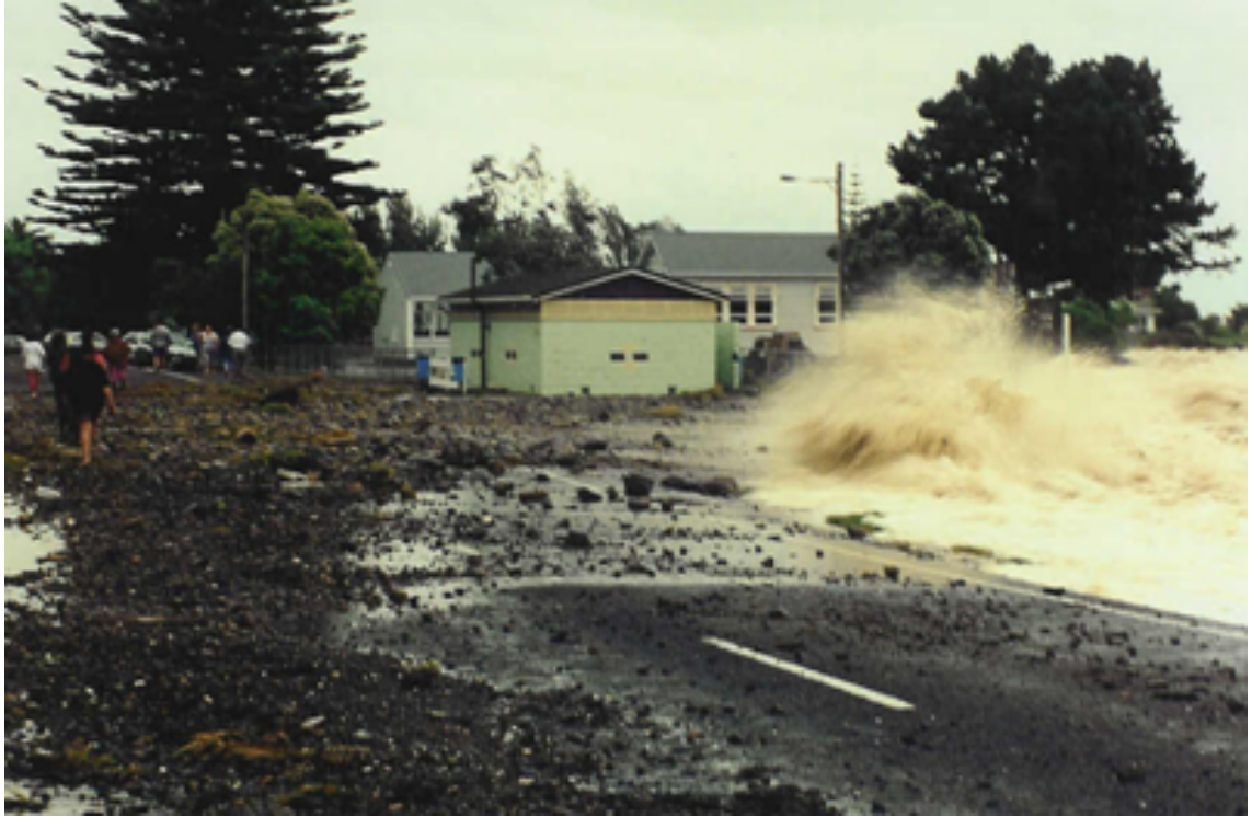
Figure 5.9: The Thames Coast Road and the Te Puru School (looking south) after the weather bomb in 2002 (photo by Civil Defence, Thames).
