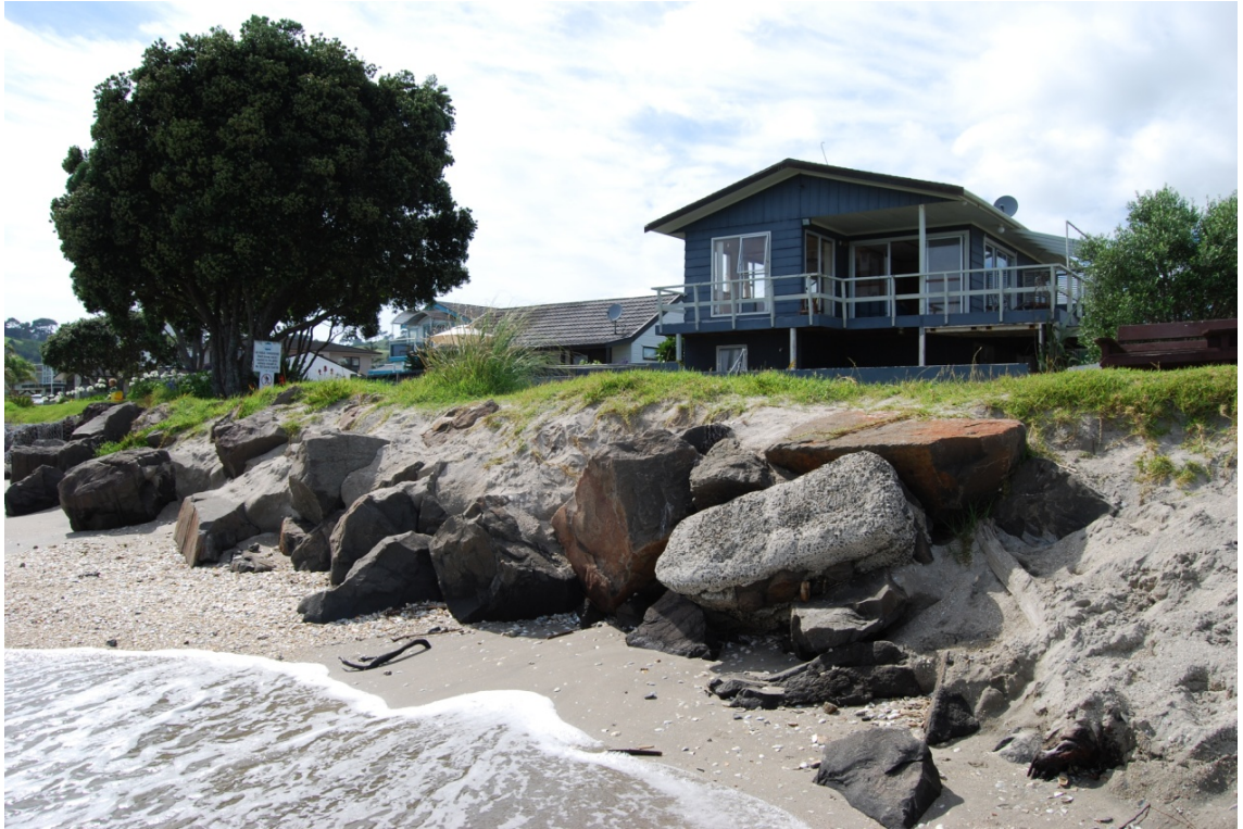
Figure 6.16: Beachfront property owners have dumped all kinds of rocks in desperate attempts to decelerate coastal erosion such as here at Cooks Beach (photo by author, 2012).
