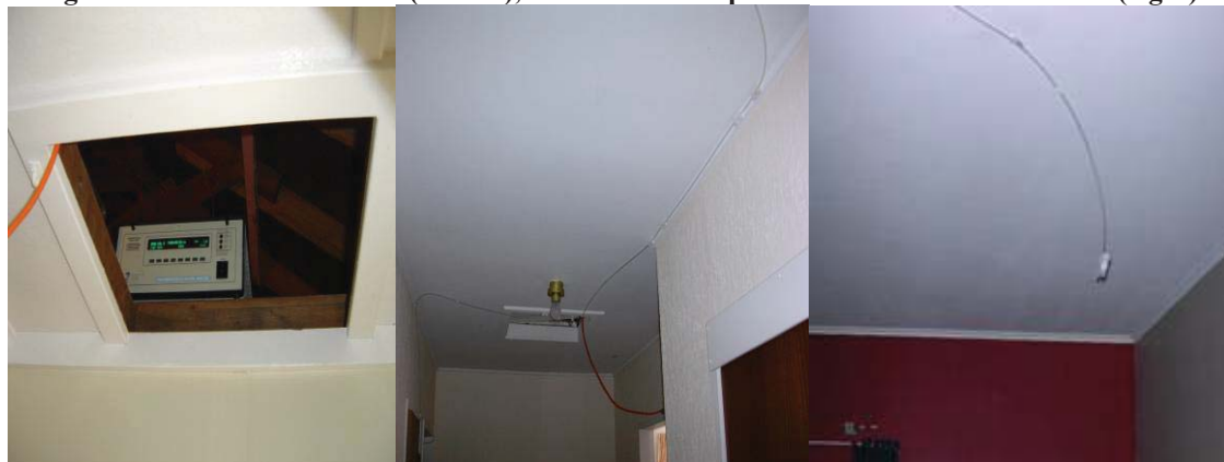
Figure 3.5: NO 2 analyser located in the roof cavity (left), tubing running from the roof cavity to the living room and to the bedroom (middle), tube end with a passive diffusion tube attached (right).
