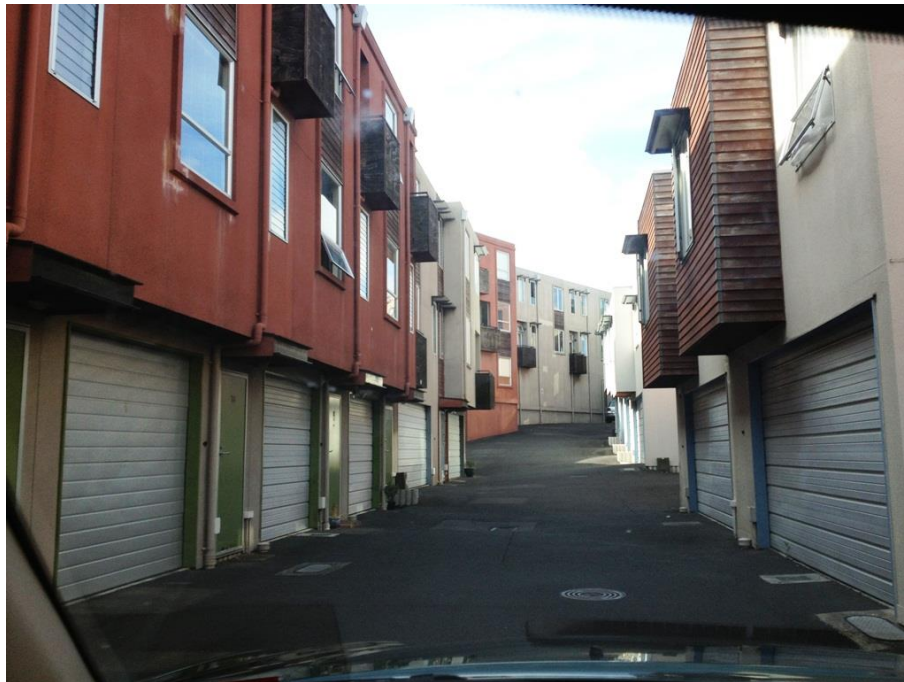
Figure 7. Poor quality and leaky townhouses (Mt. Eden)
