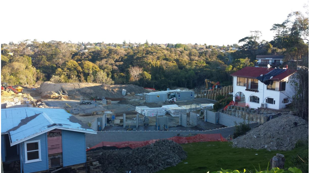
Figure 22. Development site before and during construction (photographs: author)
