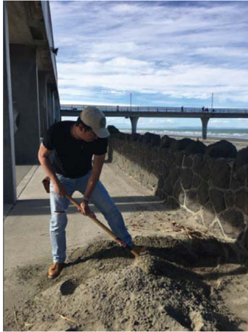
Clearing sand in order to even out the ground
