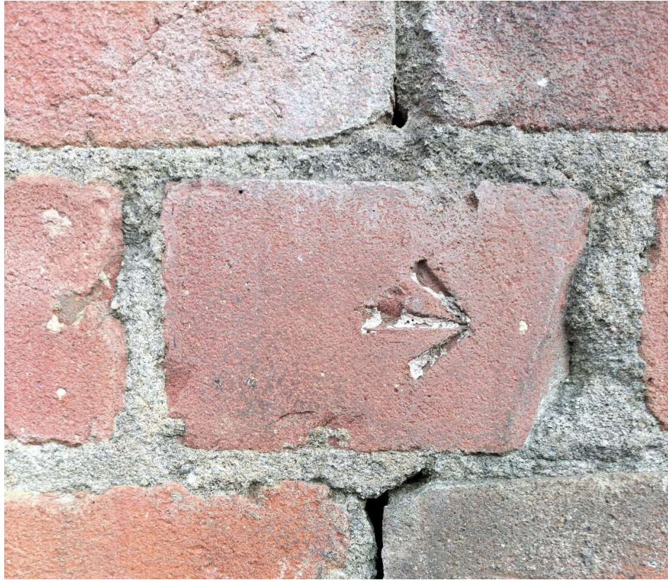
Figure 11. Tasman Street wall, detail. Te Whanganui-a-Tara, 2024.
