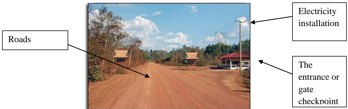
Photo 5.5 Road improvement and electricity installation in Kiet Ngong Village, Lao PDR
