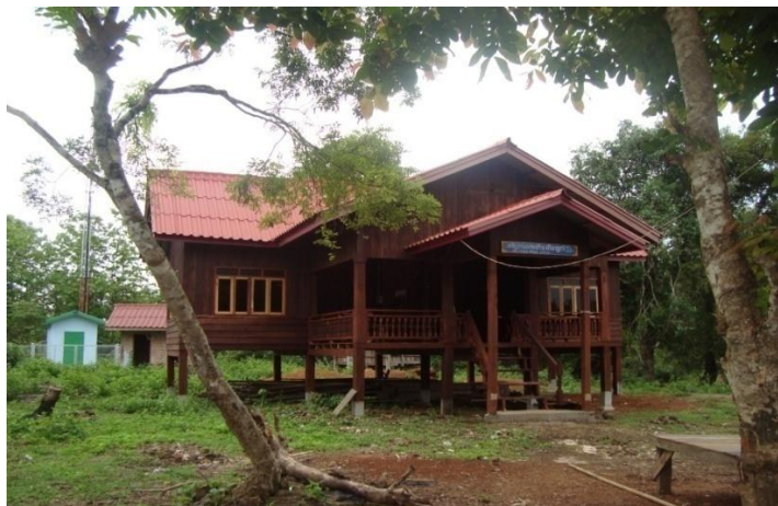
Photo 5.6 The new village office of Kiet Ngong
