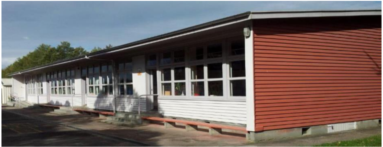
Figure 5.13: Front View (Avalon Block)
