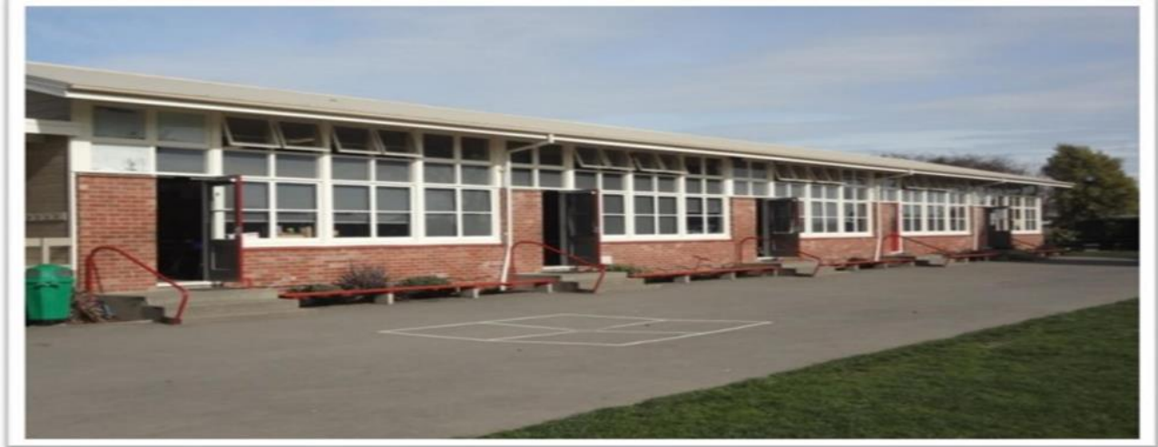
Figure 5.15: Front View (Canterbury Block)
