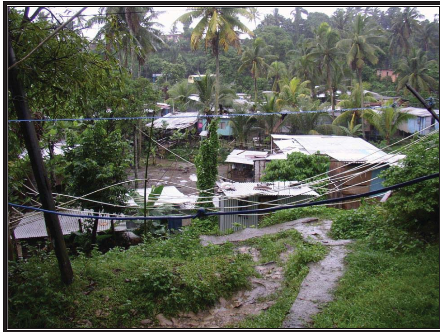
Photograph 5A: Haphazard Water & Power Connections
