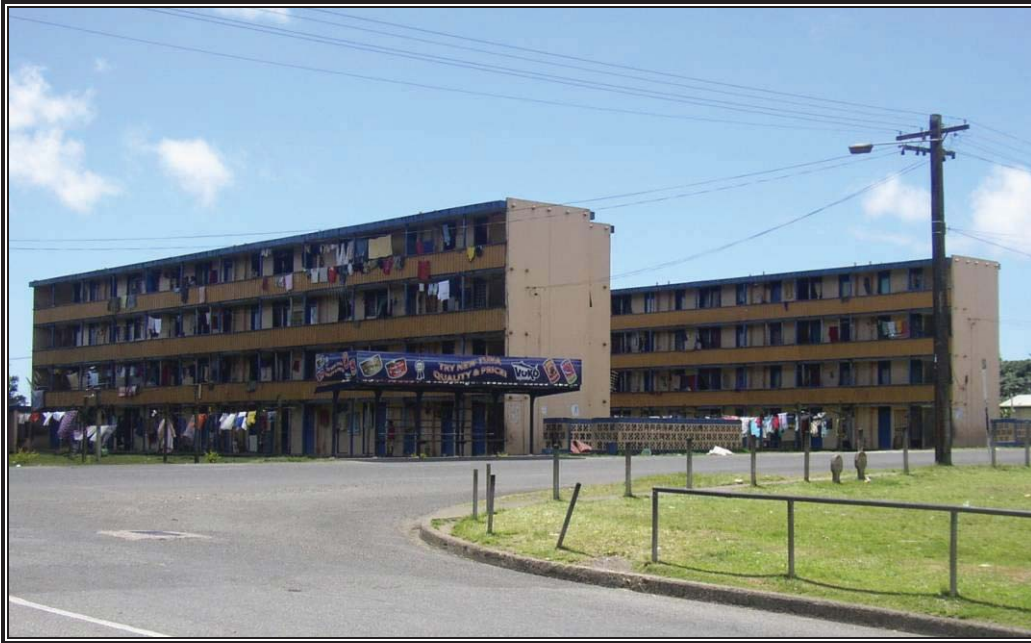
(The occupiers evicted, these flats were demolished in October 2008. Yates, June 2008)
